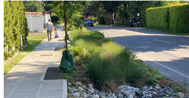
Natural drainage systems use plants and special soils to improve drainage and water quality. This image shows one possible concept for improvements on 17th Ave NW.
