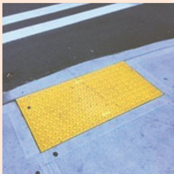
A brand-new curb ramp with its signature yellow panel and nubby texture
