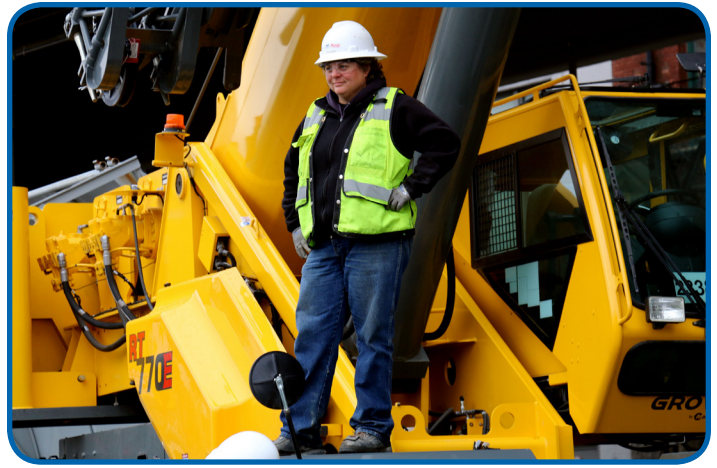
At 13 percent, women on the Seawall are working nearly three times the percentage of hours compared to past City projects.
