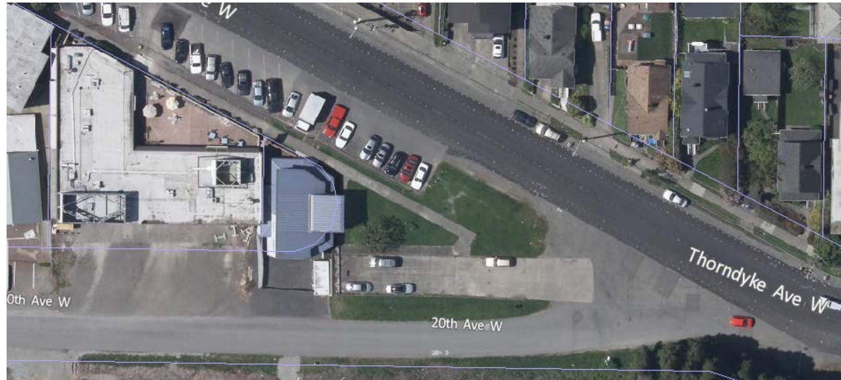
20 th Ave W – Minor Industrial Access
